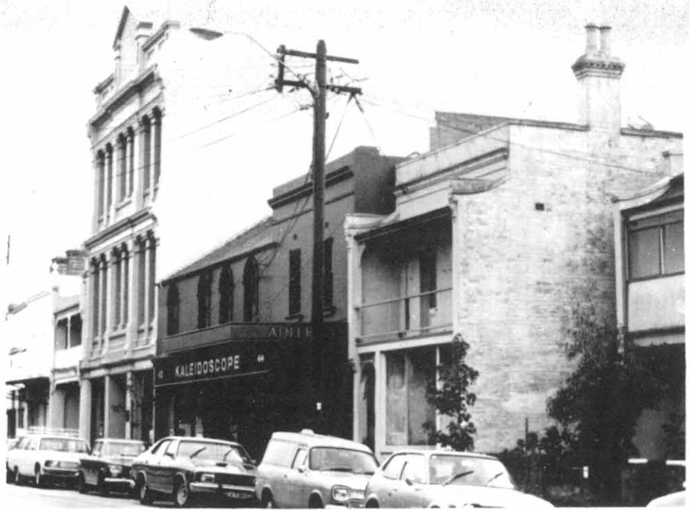
The group of properties at 34-48 Queen Street, dominated by Queen Street Galleries, which have recently been given a classification by the National Trust. All have been restored in the past 10 years, with the exception of the shop nearest the cinema camera.
